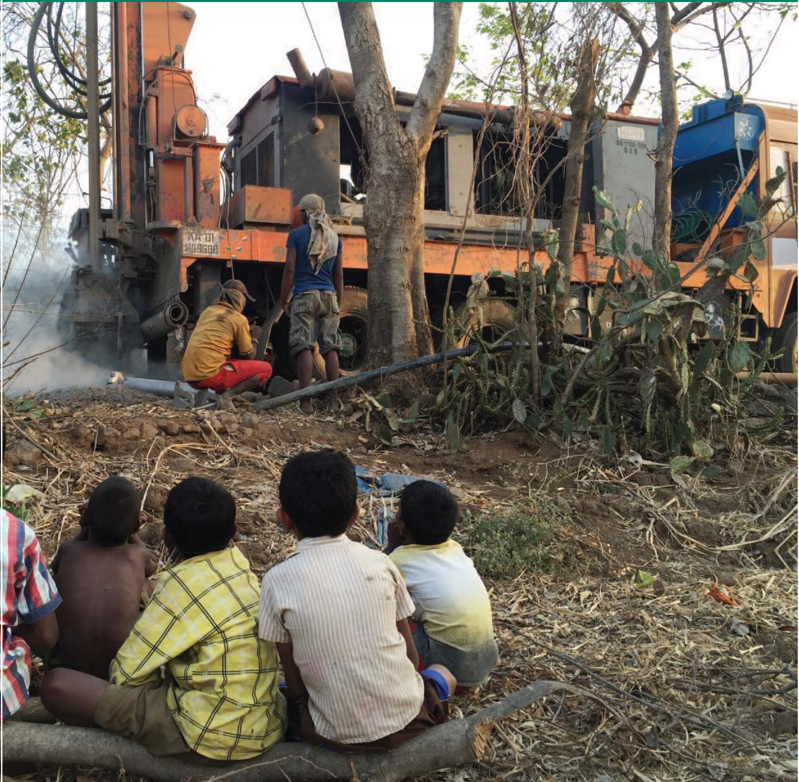
The bore well is drilled to a depth of 480 feet
